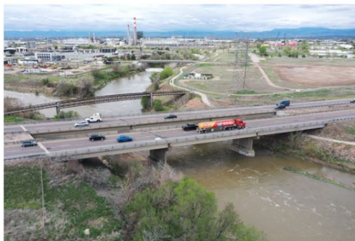
I-270 crossing the South Platte River. Pedestrian bridge for the Sand Creek Greenway trail and industrial development in the background. Facing southwest.
