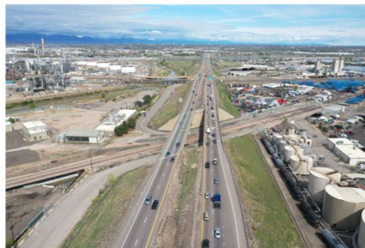
I-270 crossing over a railroad spur and 60th Avenue with industrial development surrounding the highway. Facing northwest.
